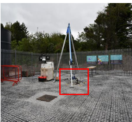
Previous borehole at United Downs under a tripod in an existing industrial site
