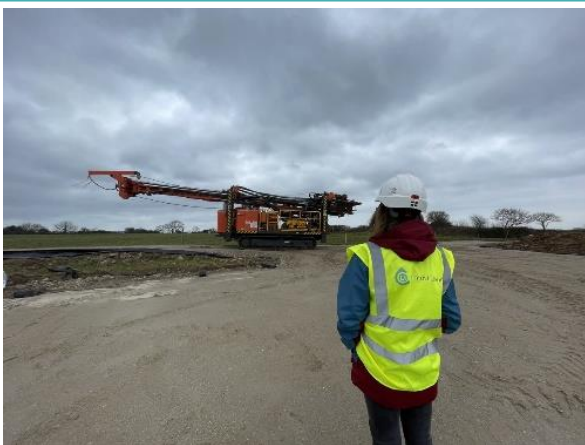
The drill rig used at Twelveheads is now at Blackwater
