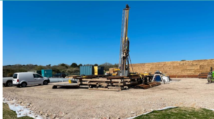
Drill rig at Blackwater with straw bale noise mitigation
